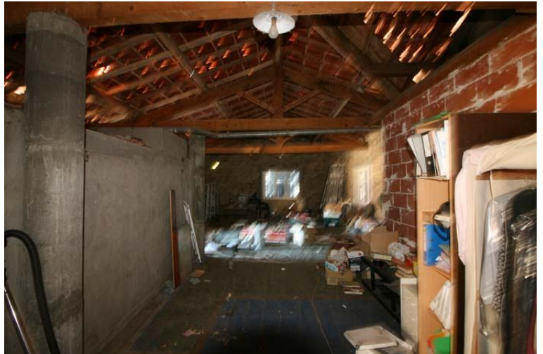
Large convertible area at first floor level
